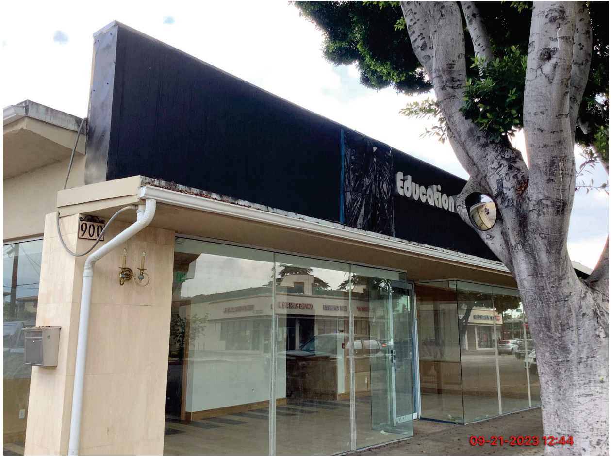
FRONT OF BUILDING
